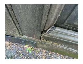
7. **Ironmongery issues:** The historic and possibly unique ironmongery is in a poor state – some of it is broken and no longer functioning and some is damaged and detached.
