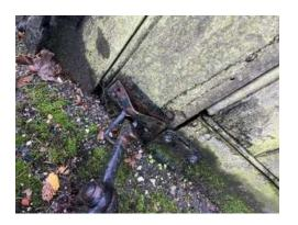
8. **Missing bollard:** One of the protective bollards is no longer there.
