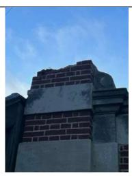
4. **Delapidation of remaining urn:** The surviving urn embellishment has a crack in it and should be looked at asap.
