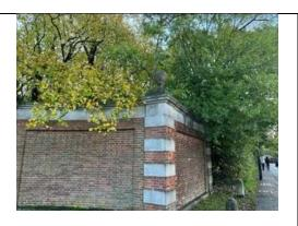
2. Impact damage to structure: The gate suffers from vehicle impact damage and is currently in a damaged state in several areas. One of the main gate pillars is missing its capping and urn embellishment as a result of the most recent collision.
