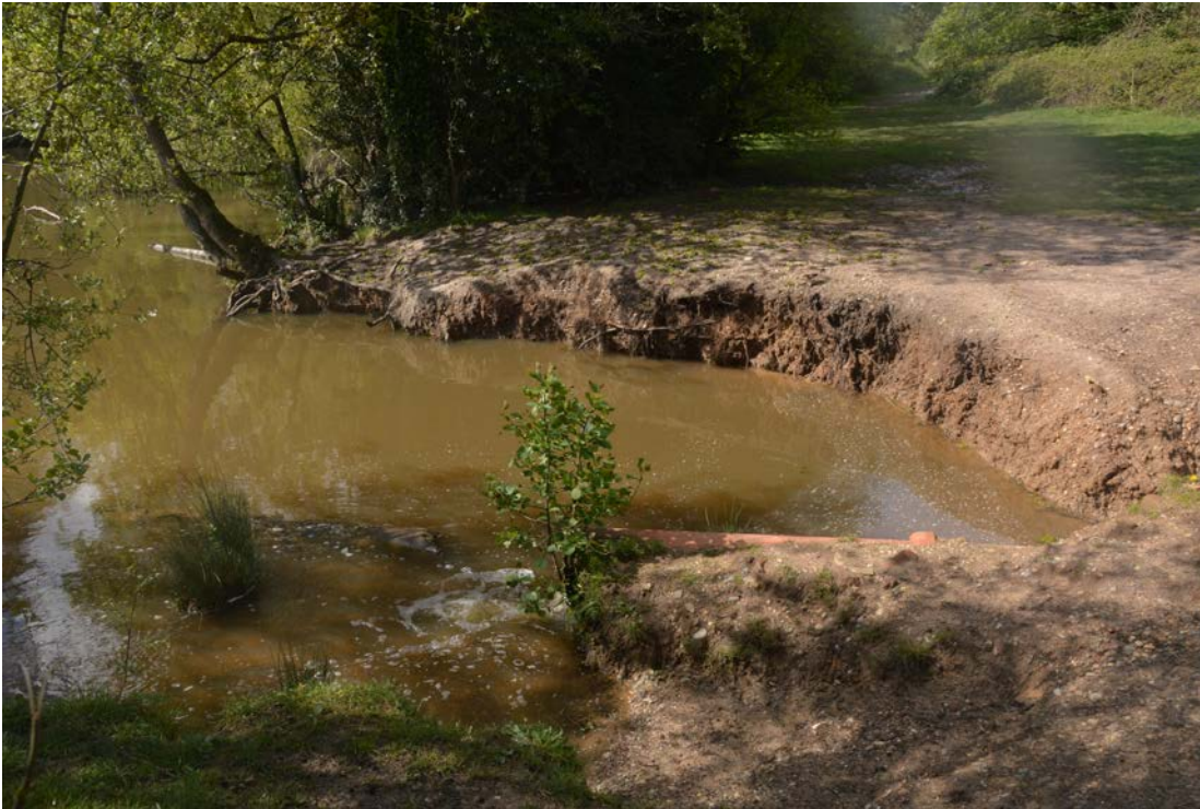
Figure 10.1 - This is the worst case of erosion of the edge, where erosion around an outfall has been accelerated by wave action.
