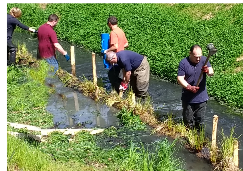
Community event at Firs Farm creating a vegetated river bank support using natural materials.
